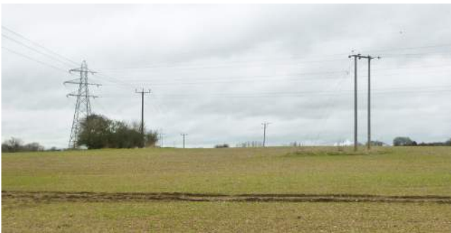
132kV, 33kV and 11kV overhead powerlines
